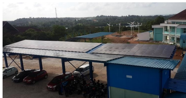
Figure 7. Solar Module Carport in UMRAH
