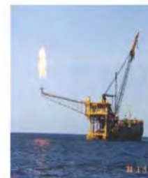
Photo: Rang Dong Oil Field Associated Gas Recovery and Utilization Project – sources: DNA Vietnam
