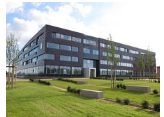
Full view on the Extension Building
